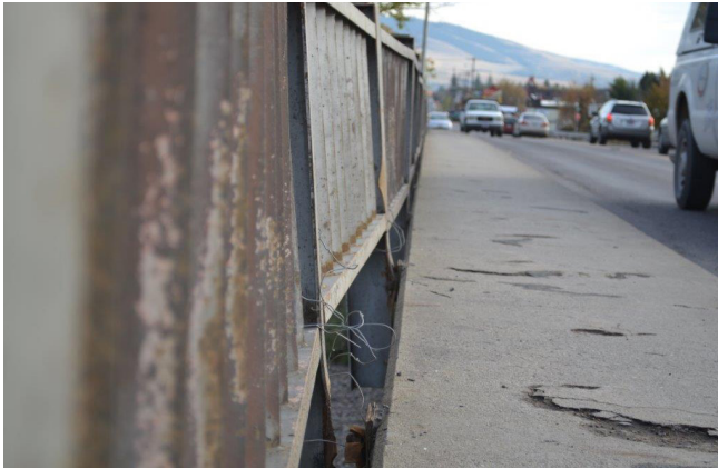
Deteriorating sidewalks on the Russell Street Bridge
